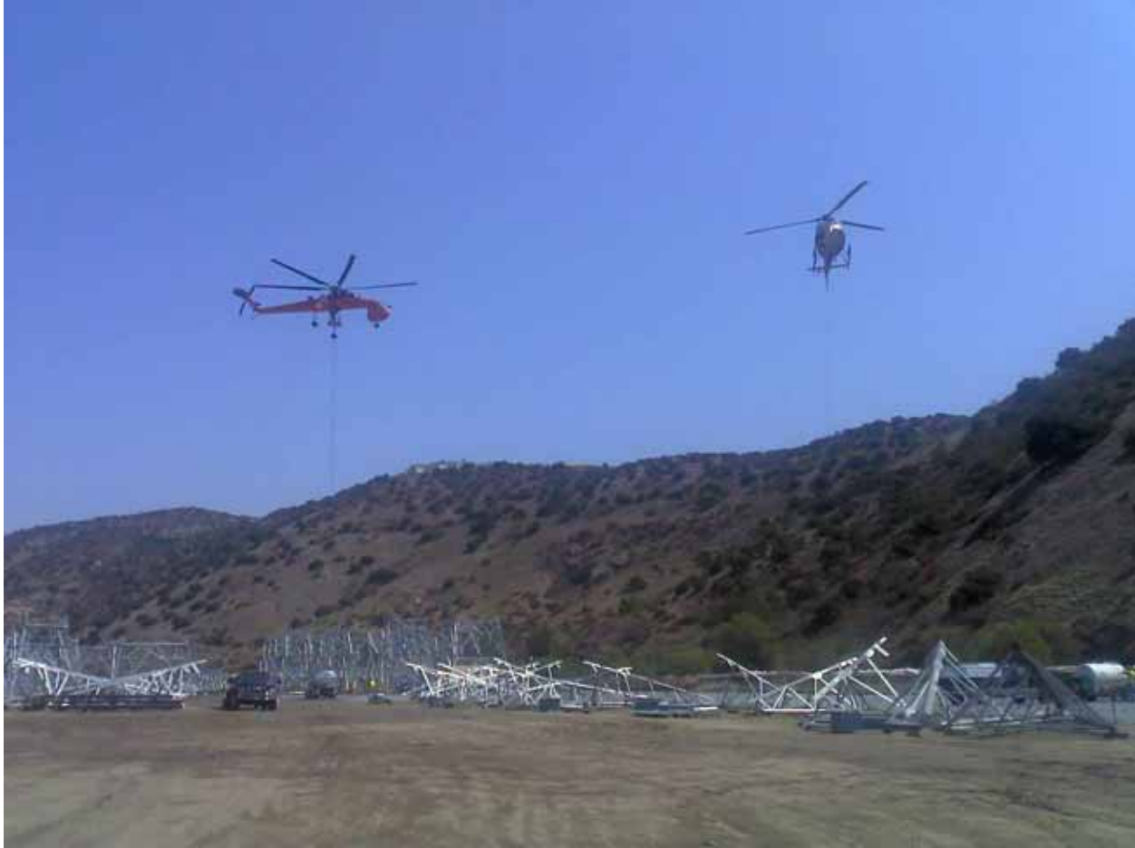
Helicopter activity at Helix Yard. Photo courtesy of Randy Burke.
