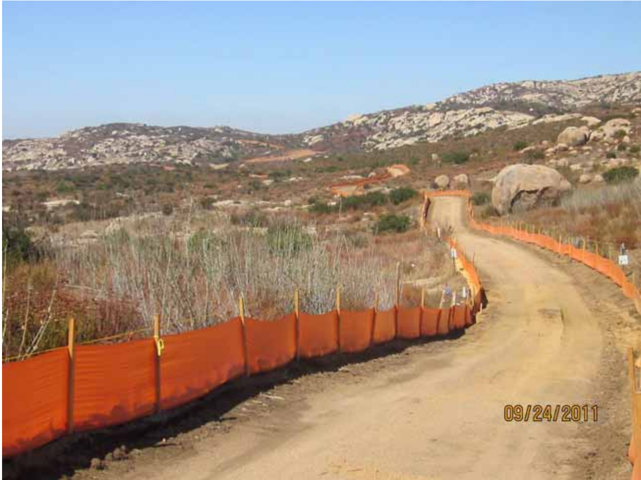
Arroyo toad fencing at Kreutzkamp. Photo courtesy of Kham Slater.
